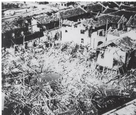
Destruction caused by incendiary bombs on the wooden structures of the Hongkou and Chapei
