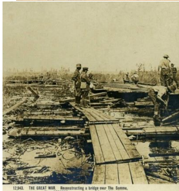
12343. THE GREAT WAR. Reconstructing a bridge over the Somme.
