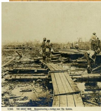
12943. THE GREAT WAR. Reconstructing a bridge over the Somme, near Villers Carbonnel.
